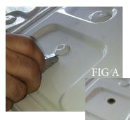
6. Once the correct mounting positions have been determined, carefully and gently run the blade along the bottom edge of the plug with an exacto knife or blade to remove the plug and access the factory mounting positions. FIG A.
