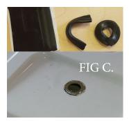
8. After the plugs have been removed and the threads cleaned, cut the buttle tape squares provided into approximately 1/4" strips. Bend the strips around forming a circle with the center opening just big enough to pass the M8 x1.25 x 35 flat socket screw through. Place around each of the factory mounting positions to be used to secure the channels. FIG C.
