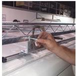
19. With the holes drilled through and the van rack assembly clamped in place, secure the van rack assembly to the supports using (2) 5/16°-18° x 2-1/4° hex head bolts, (2) 5/16° flat washers and (2) 5/16°-18 nylon locking nuts on each support. Be careful not to over tighten, doing so may cause damage to the rack or the van. FIG I.
